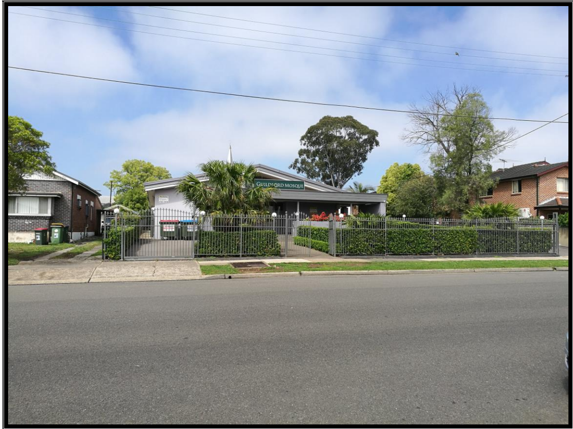
Photo 1: Existing site frontage to Mountford Avenue
